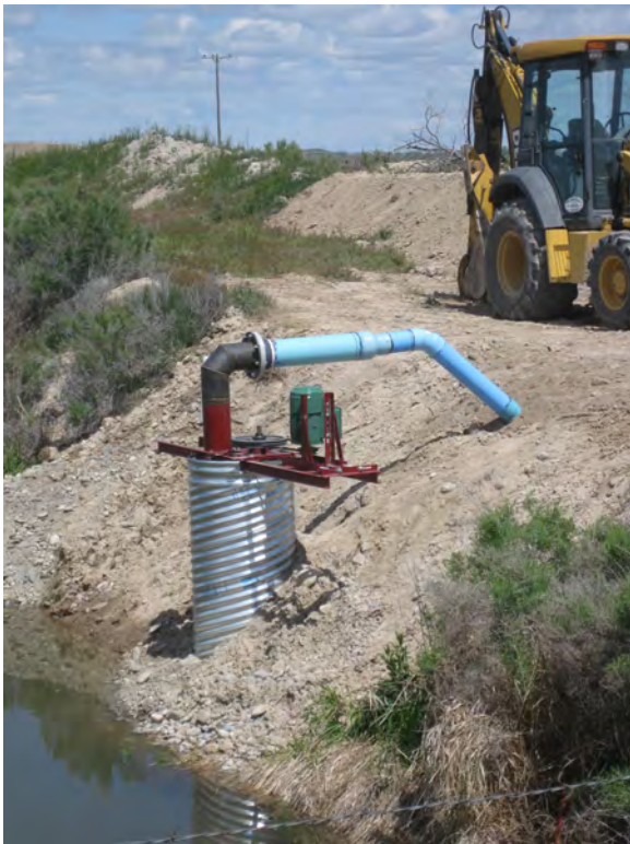
Figures 10A and 10B - Installation of the Pump and Pump Well at North Alkali Drain
