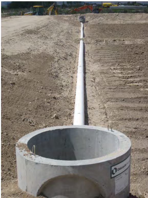
Figures 6A and 6B - Distribution Manifold at the Head of the Grow Plots
