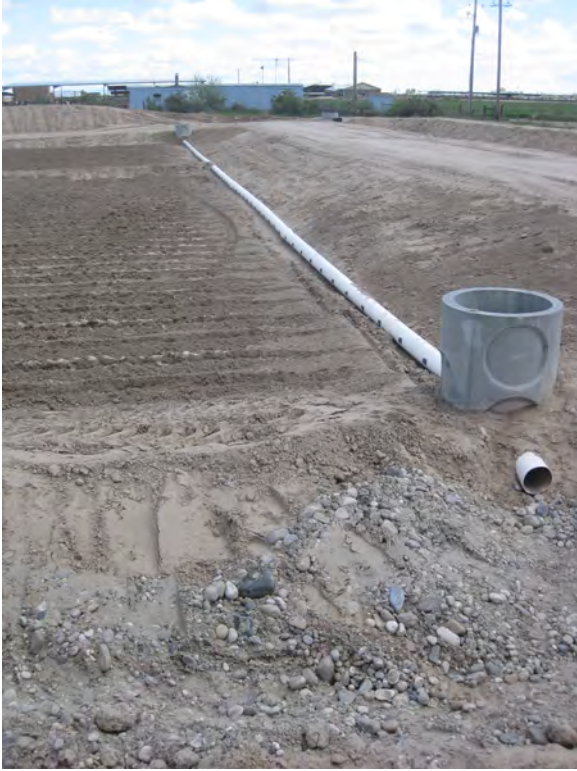
Figures 9A and 9B - Distribution Manifold, Bypass Standpipe, and Flow Measurement Device
