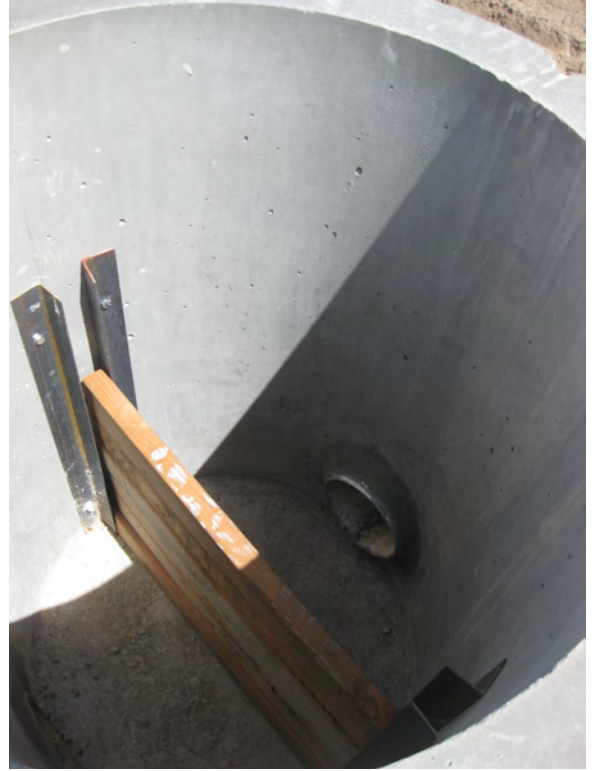
Figures 7A and 7B - Bypass Ditch and Standpipe With Boards That Portion Flows Between Ditch and Grow Plots
