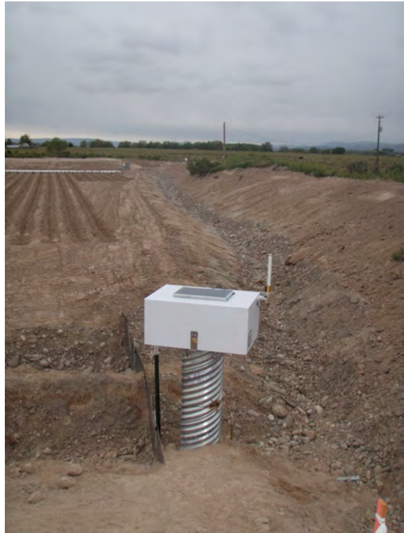
Figures 9A and 9B - Distribution Manifold, Bypass Standpipe, and Flow Measurement Device
