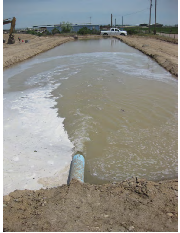
Figures 3A and 3B - Excavation and Operation of the Sedimentation Basin
