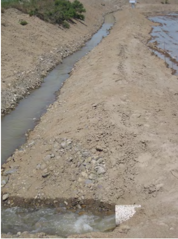
Figures 7A and 7B - Bypass Ditch and Standpipe With Boards That Portion Flows Between Ditch and Grow Plots
